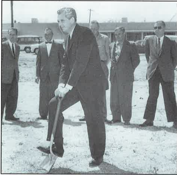
Groundbreaking for the Cooper Cinerama Theatre on Colorado Boulevard in Denver, Colorado. Left to right: Unknown; Unknown; Kenneth Anderson, president; Cecil Hart, construction superintendent, Berglund-Cherne Company; Buck Winans, sound engineer; unknown. Denver Post Photo.
